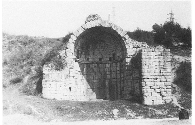
(c) Apse at east end of bridge.
