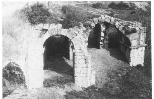
(e) First phase vaults from west.
